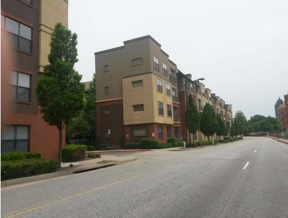
Mid-rise apartments at Atlantic Station in Atlanta, GA yield about 20 homes per acre, making nearby walkable commercial areas more vibrant and successful.
